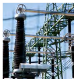
Electrical generation, transmission, distribution, installation & maintenance
