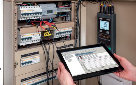
Installing an energy logger on equipment that uses large amounts of electricity can provide clear and revealing information about energy use
